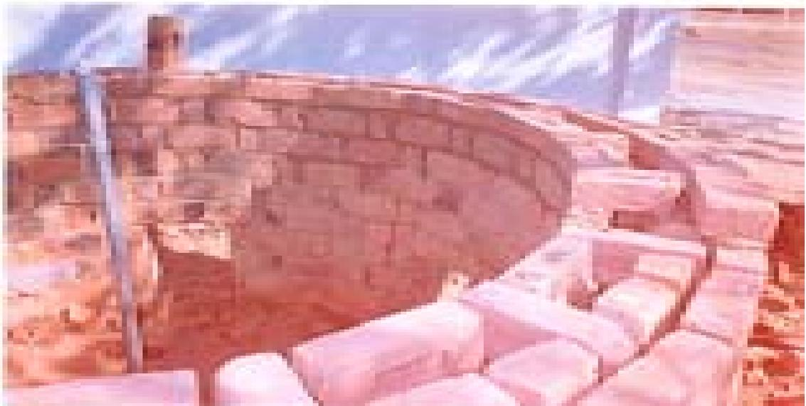
Figure 2c. Kiln wall during construction
