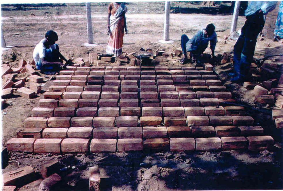
Figure 3: Kiln floor during construction
